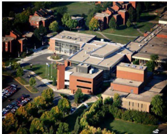
Figure 2 Arial image of Southwest Minnesota State University in the Fall)
